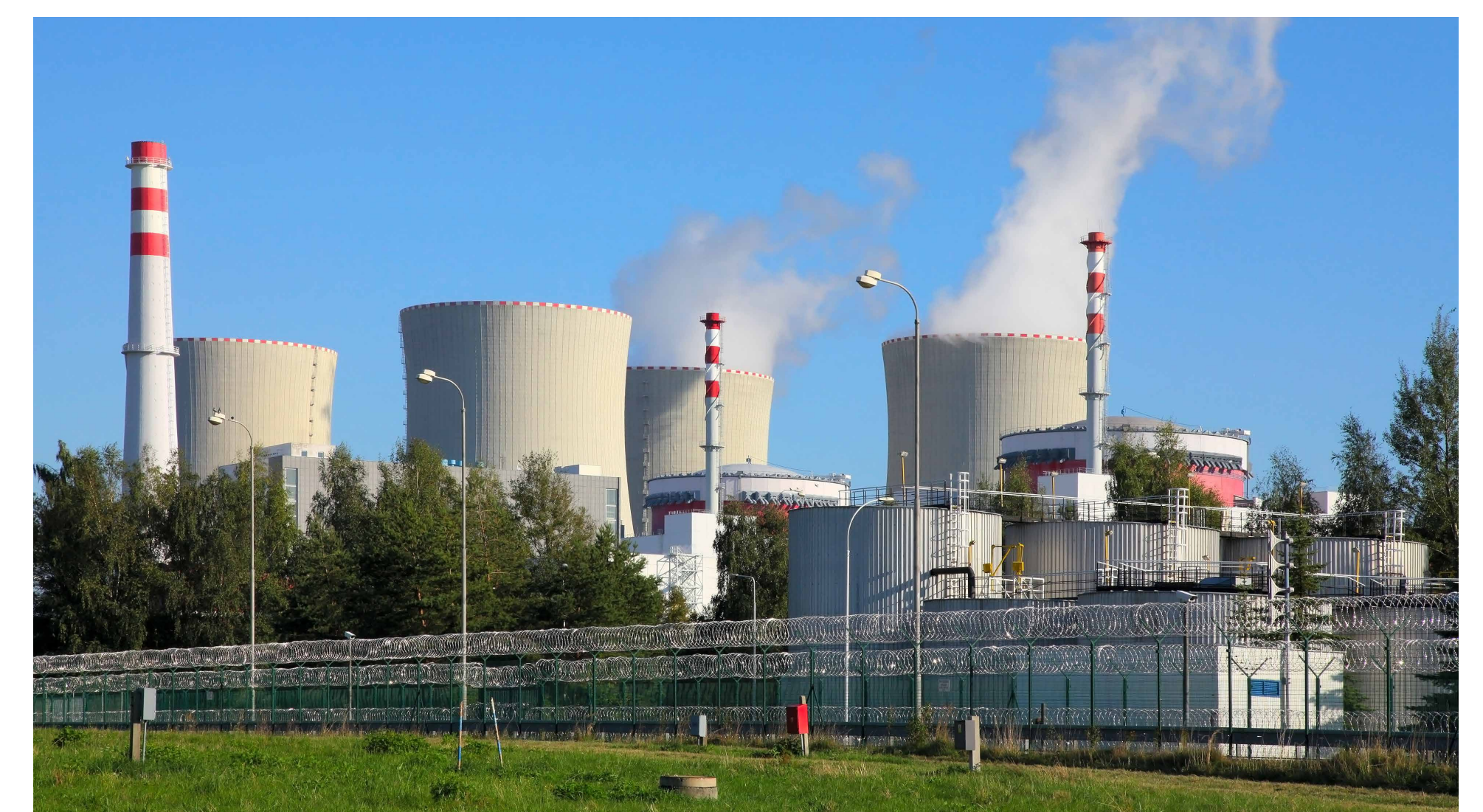
Temelin Nuclear Power Plant in Czech Republic
