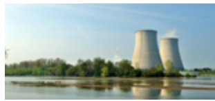
Nuclear access control
