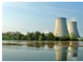
Ring monitoring for nuclear facilities
