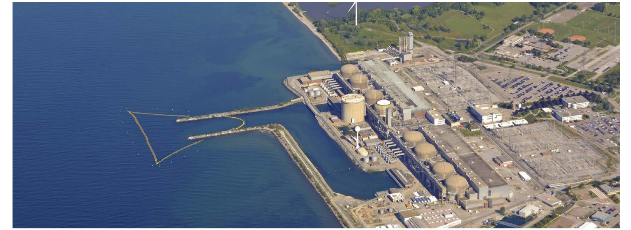
Bruce Power nuclear power plant (BP NPP) in Ontario, Canada
